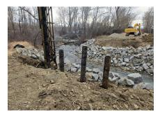
Since the project was let to bid and contract documents were executed with Battle Ridge Construction, the old bridge has been removed, riprap has been installed, piles have been driven for both abutments and concrete has been poured for bridge cap. The construction team is awaiting delivery of the bridge superstructure and the project is slated to be complete by July 25th, 2025 (or sooner).
