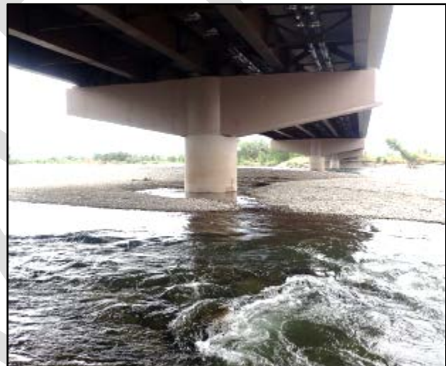
Figure 10: Drilled Shaft Foundation
