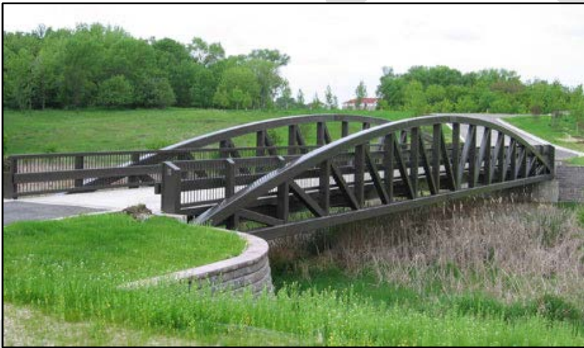
Figure 7: Keystone Truss
