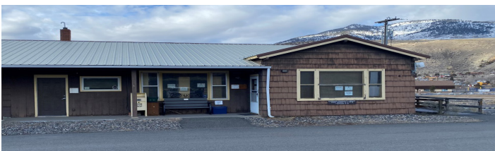
Figure 7: Gardiner Depot Building
