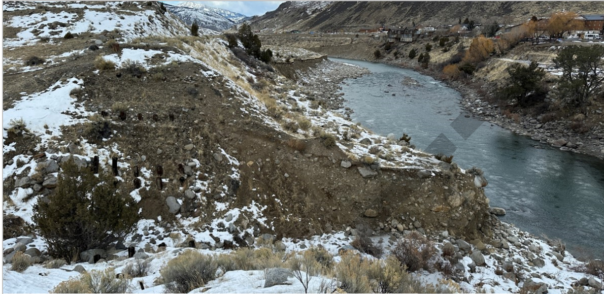
Figure 4. Photo of the Pinedale flood deposits taken during a site reconnaissance.
