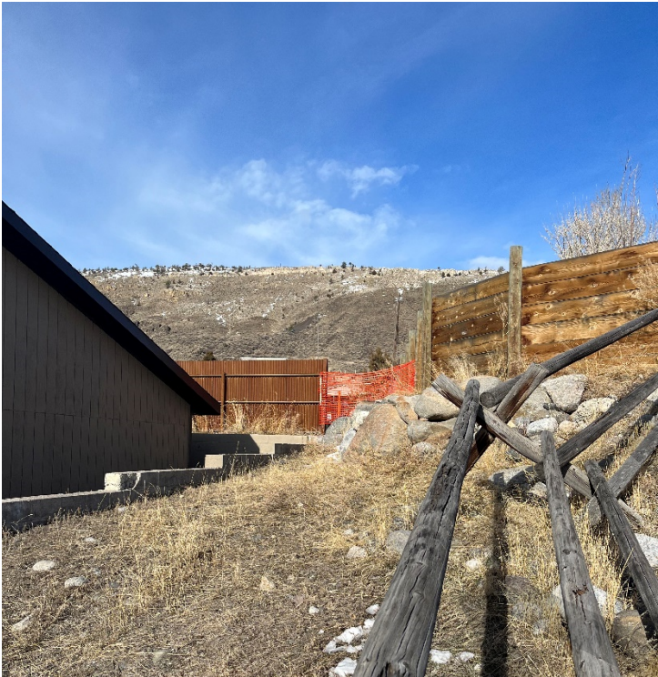
Figure 8. South connection to Delaware North Property.
