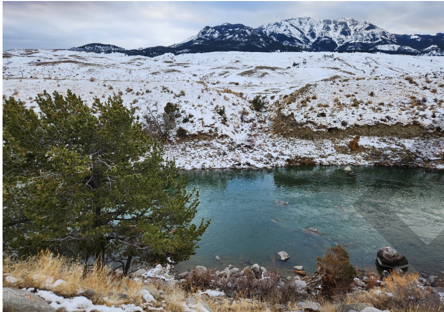
Figure 11. Noticeable Erosion/Scour on South Bank of the Yellowstone River.
