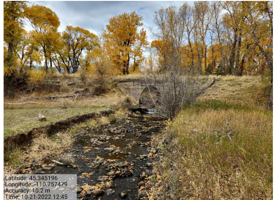
Photo 4. Fridley Creek, large railroad arch culvert
