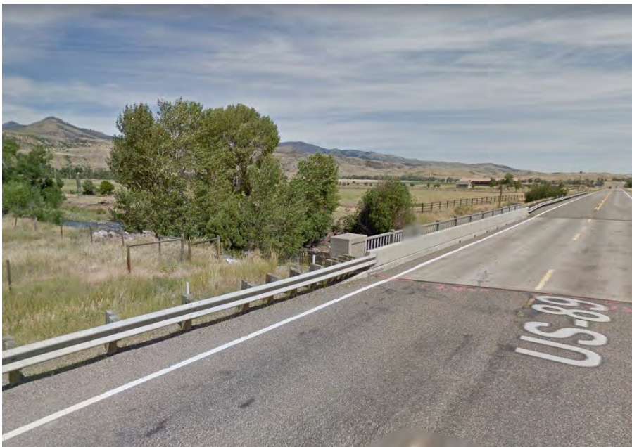
Photo 3. Big Creek bridge area.
