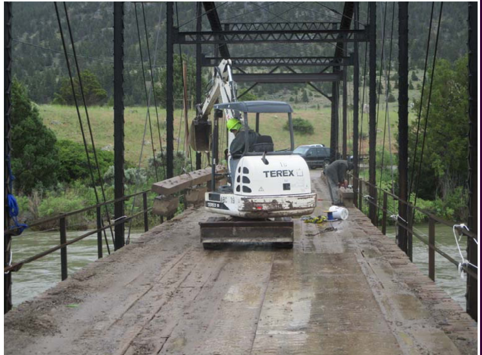
Removing the existing curb blocks and railing for reuse.
