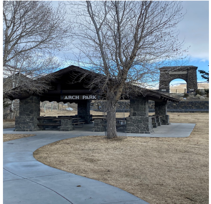
Figure 10: Arch Park in Gardiner
